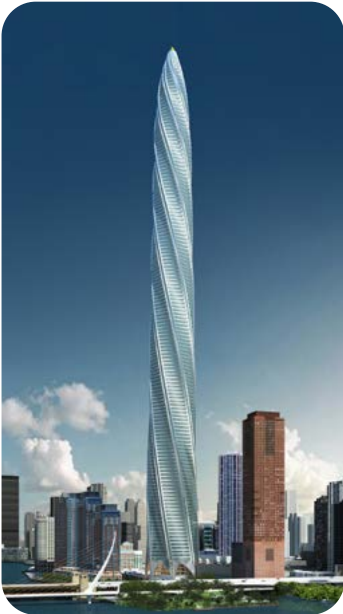
The Chicago Spire, with Santiago Calatrava Architects, 2000ft (609M) 1200 Unit Residential Tower Project Architect With P+W
