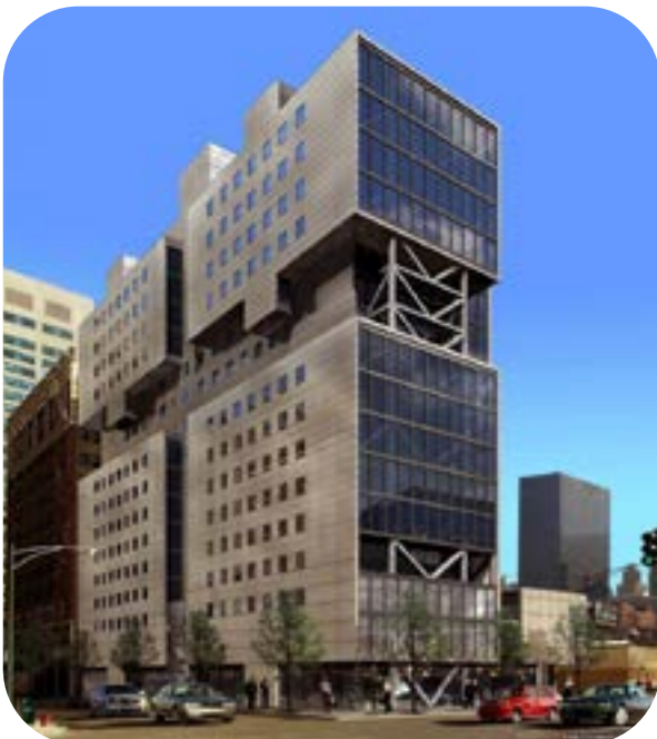
Godfrey Hotel, Chicago Illinois, 18 story hotel staggered steel truss structure Project Architect With VDTA
