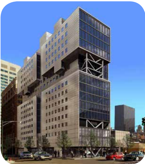
Godfrey Hotel, Chicago Illinois, w/VDTA 18 story hotel staggered steel truss structure Project Architect
